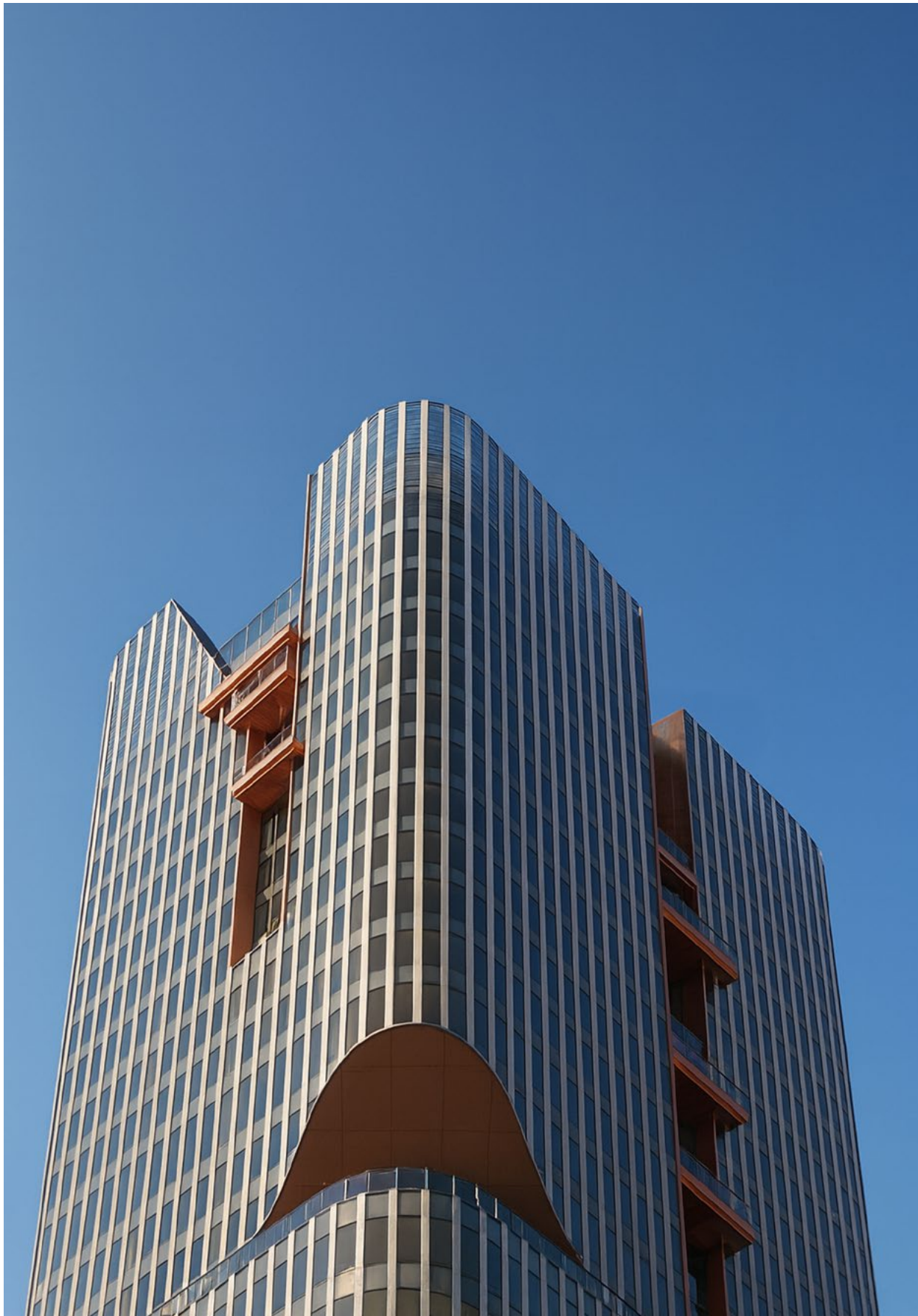
Undisclosed project - Atchain
