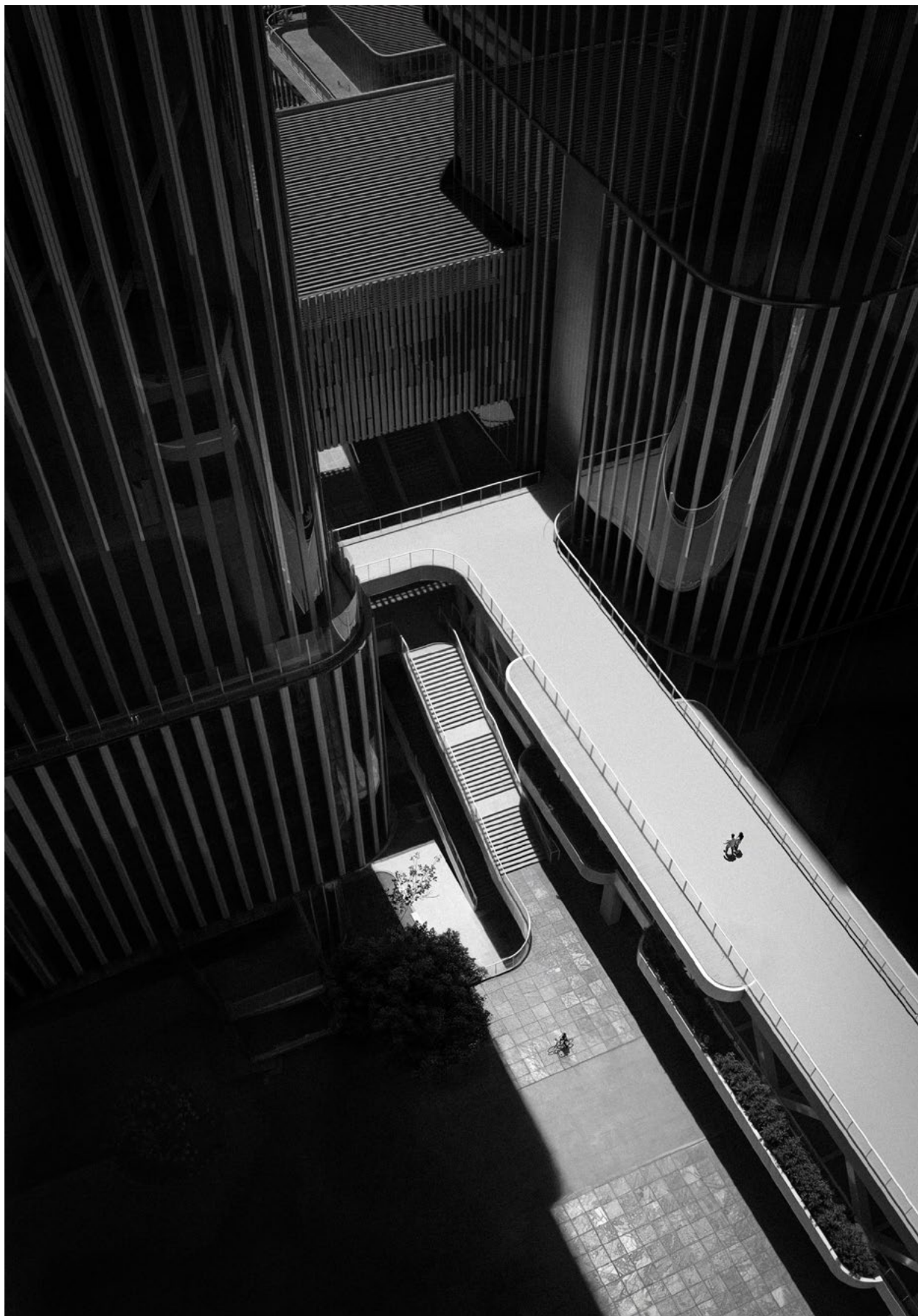
Undisclosed project - Atchain
