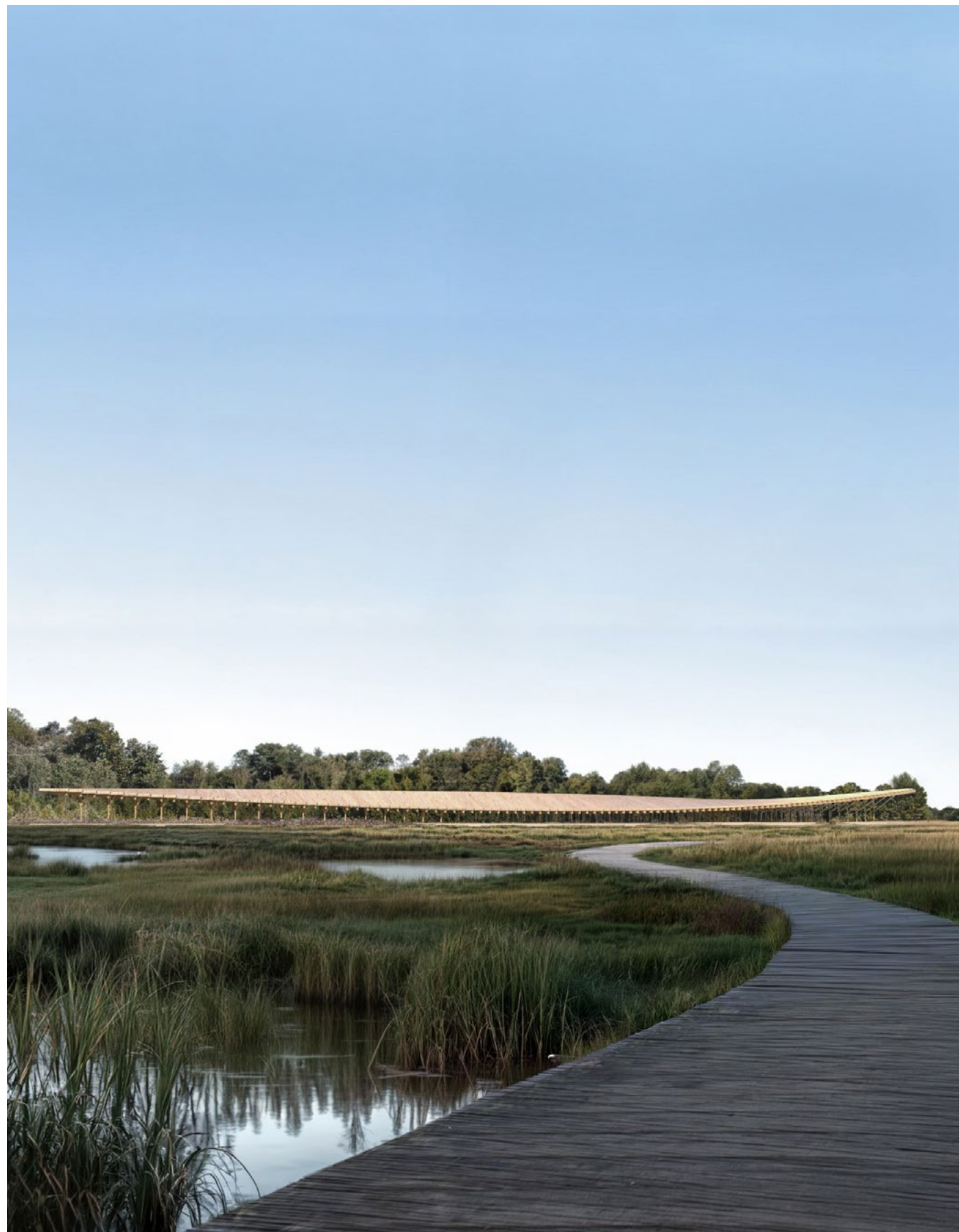
Visitor Center at Butrint - Kengo Kuma and Associates
